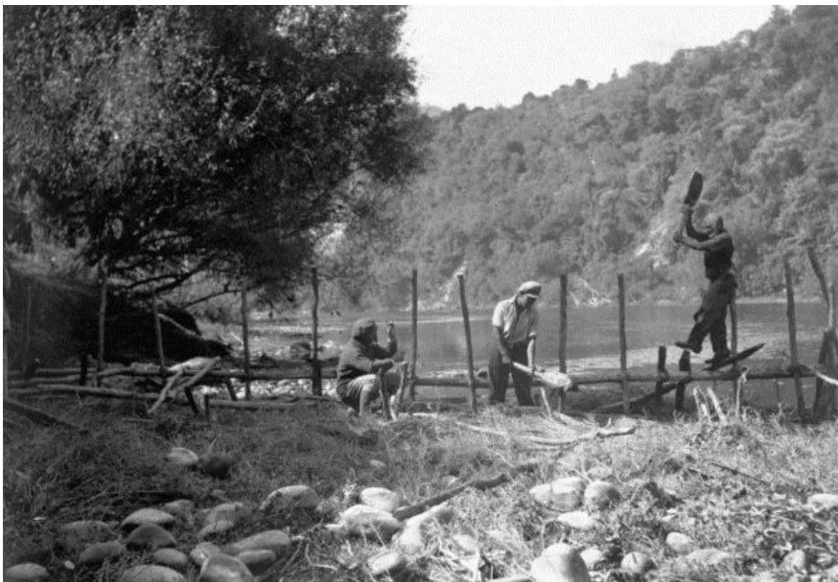
Figure 6: Making a lamprey weir at Hiruhārama, Whanganui River (Photo: JI McDonald 1865–1935. Ref: PAColl-1430-30. Alexander Turnbull Library, Wellington, New Zealand ( http://natlib.govt.nz/records/22912256 )).
